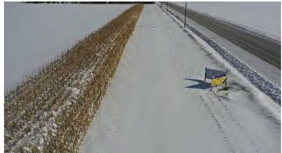
View of standing rows of corn that make up a living snow fence along Kishwaukee Valley Road in McHenry County
