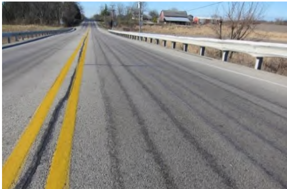
Striping on road from liquid “anti-icing” application
