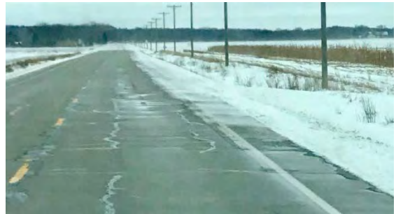
View of bare pavement on roadway next to “living snow fence” of standing corn rows in McHenry County
